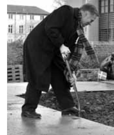
Professor Niels Elers Koch made the first sod cut to the new building.
